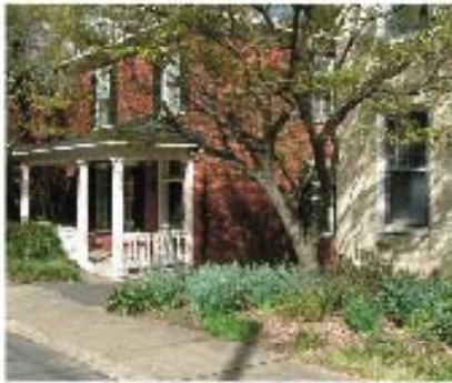
1st St. 14' Front SB w/ 6'-8" encroachment
