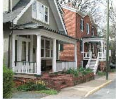
1st St. N.E.-10'-4" Front SB w/ 6'-6" encroachment
